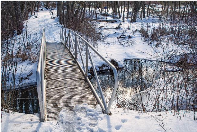
2 The current bridge over Beaver Brook.
