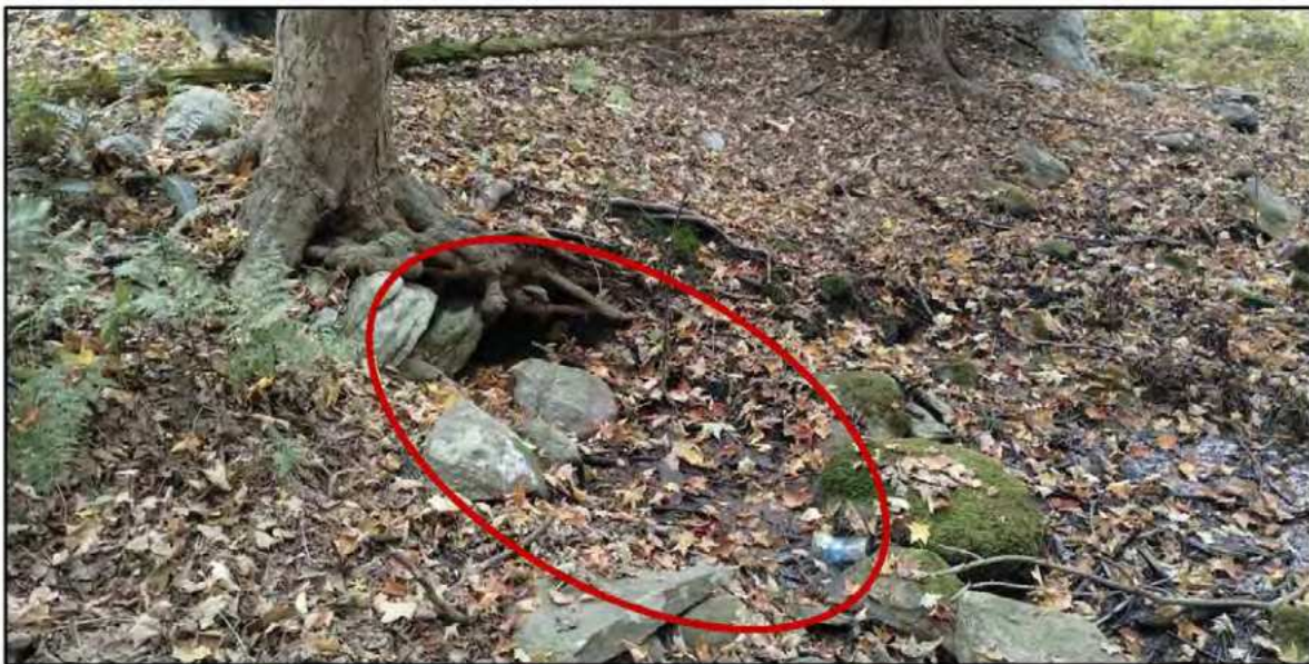
Photo 11 – Seep located beneath tree on eastern slope parallel to access road.
