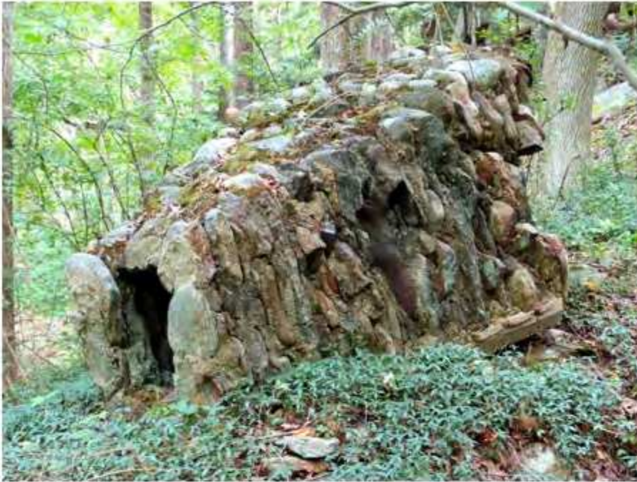
Collapsed Chimney
