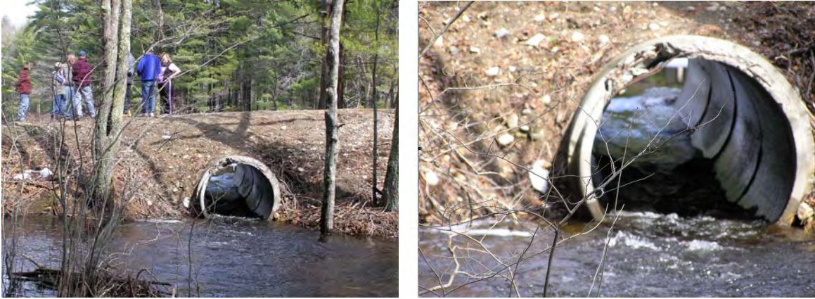
Figure 6. Out-flow of Jerry's Swamp is through 3-4' concrete pipe that passes beneath abandoned rail-bed.
