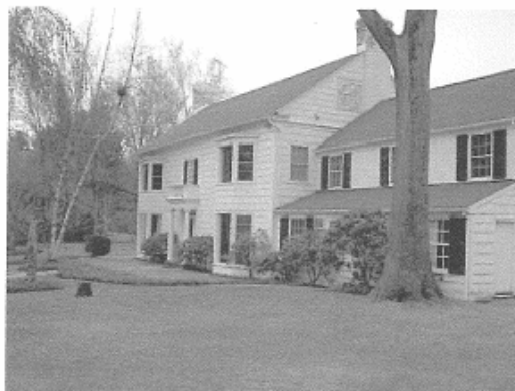
Figure 6 - House to be removed according to proposal.
