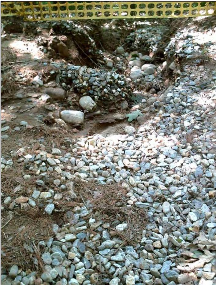
In this photograph, the gravel road immediately to the east of the to-be-mitigated wetland runs parallel with the orange fence. This washout is perpendicular to the fence and thus is headed directly downhill into the pond. It brings with it substantial sediments. This location is underlain by sand and gravel so that any surface disturbance will easily transform into sediment laden runoff, the results of which were readily apparent in the pond.
