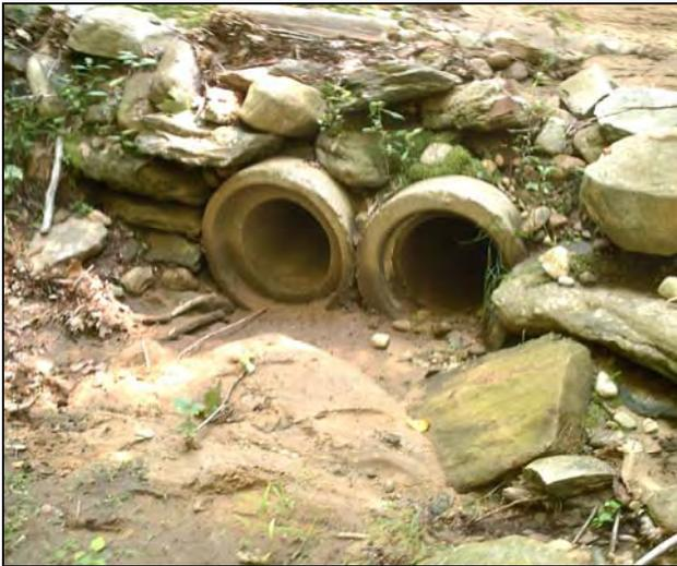
In this series of photos the west-to-east, well defined, intermittent stream course passes under the old road via twin concrete pipe culverts. Actually, the pipe on the left (north) is clear for passing water but the pipe on the right (as seen below) is clogged. This clog forces all the flow to the pipe on the left and most likely passes it with increased velocity. That could have downstream impacts of sediment in the watercourses.
