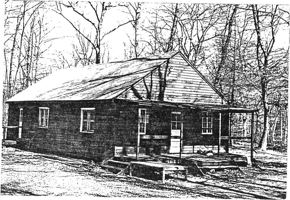
EXISTING ADMINISTRATION BUILDING
