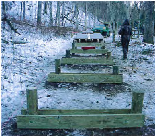
Fence posts and salt treated lumber were used to construct the supports and framing for the boardwalk
