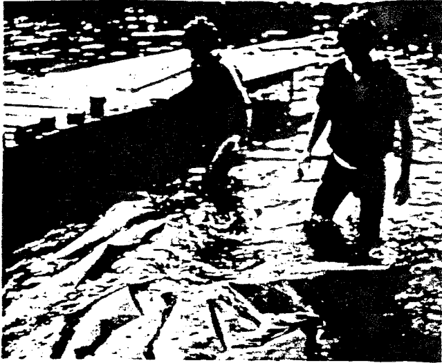
Smothering material is "walked down" and smoothed out prior to anchoring with pins, rocks or bricks.
